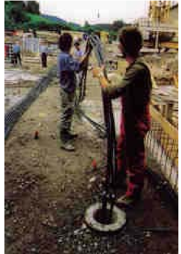
Energy piles installation
