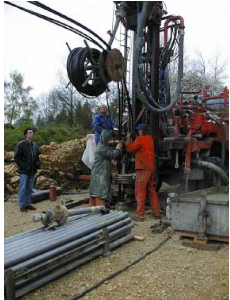
BHE drilling and installation
