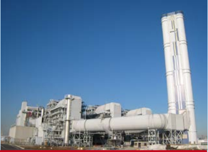
Combined Cycle Power Plant
