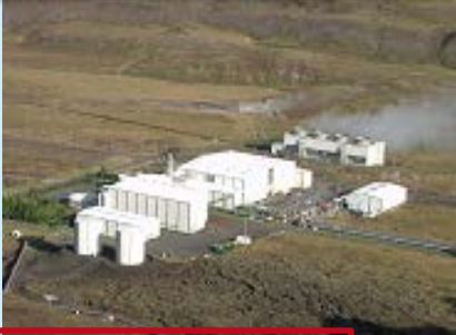
Geothermal Power Plant
