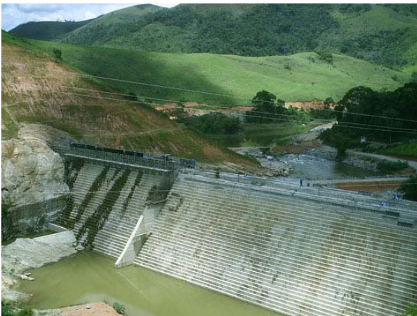
Santa Rosa Power Plant – RJ – 30 MW
