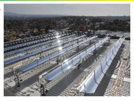
"Because we need to focus exactly on one point (the solar tube), the tracking needs to be very accurate. Yokogawa's HXS10 solar controller makes this possible."
