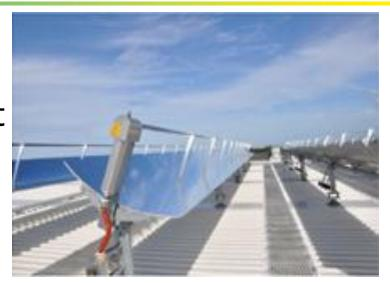
The 345 square metre 'PolyTrough 1200' solar field is mounted on a rooftop above a cinema complex. The chiller uses the heat from the solar field and a concentrated salt solution in which water gets absorbed and re-absorbed, exchanging heat in the process.
