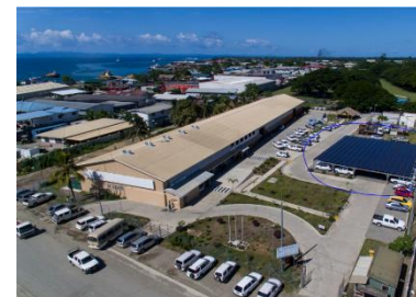
50kWp On-grid Solar PV – HEAD OFFICE RANADI
