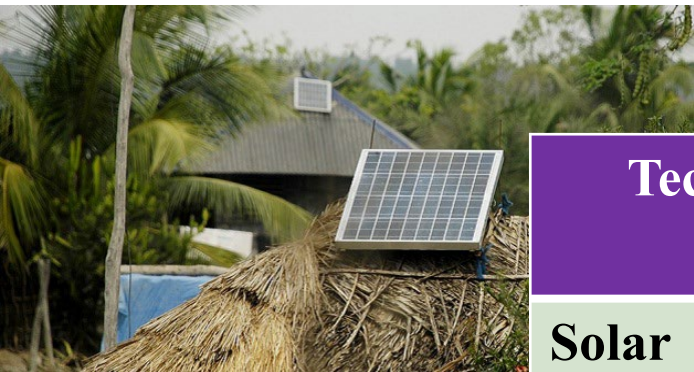
Solar Home System
