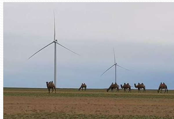
“Tsetsii” WPP Installed capacity-50 MW 2017 year
