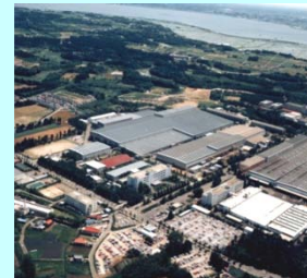
Hitachi Plant Technologies, Co., Ltd
