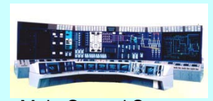
Main Control System
