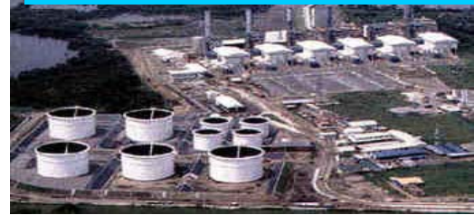
1,000 MW Sta. Rita First Gen/ IPP
