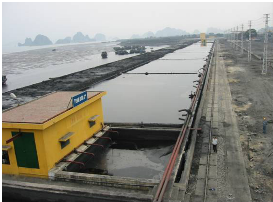
The Cuo Ong coal preparation plant, Viet Nam
