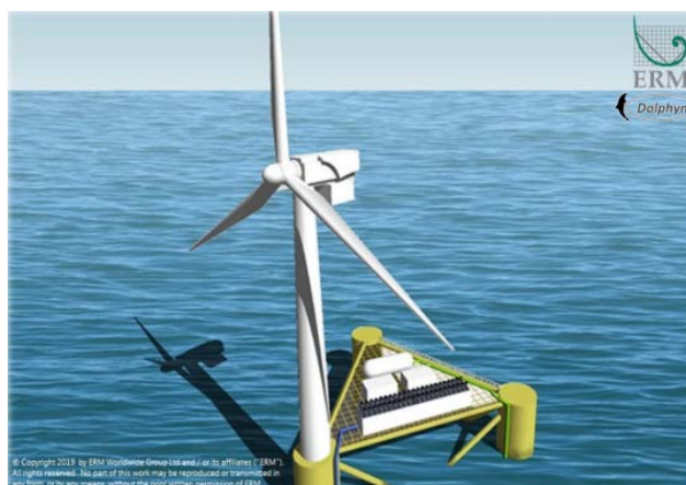
Figure 1 Floating wind farm platform designed for hydrogen production
