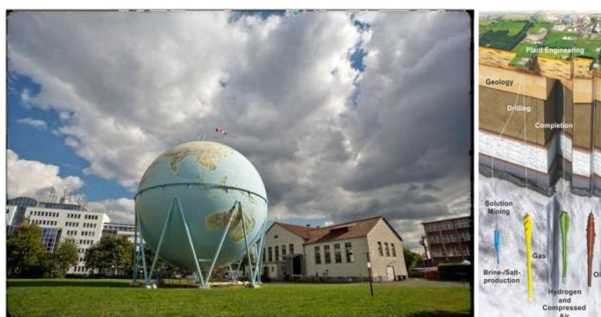
Fig. 3-5 Natural Gas Holder (left) and Underground Storage (right) in Germany
