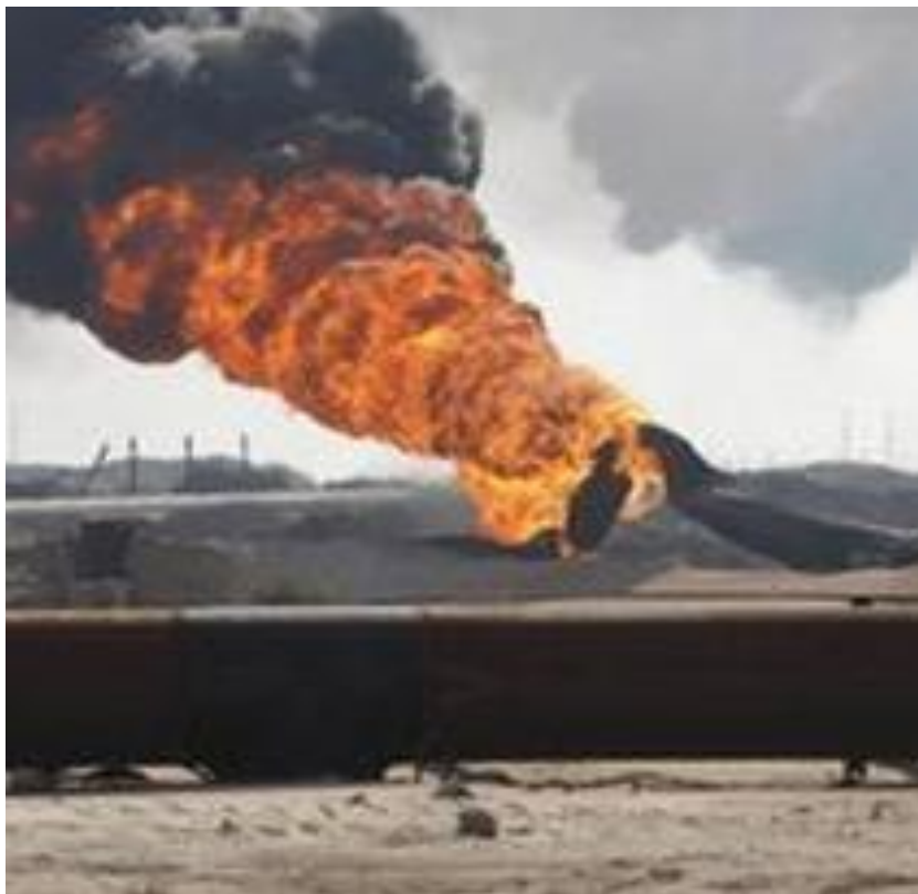
The El Arish gas pipeline after a militant attack, Egypt 2013
