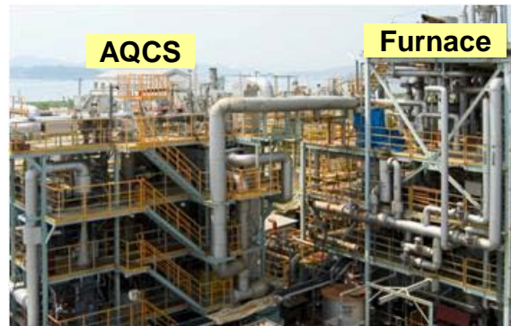
1.5MWth Test Facility
