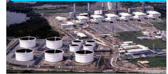
1,000 MW Sta. Rita First Gen/ IPP
