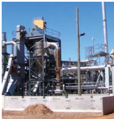
A biomass-fired power plant
