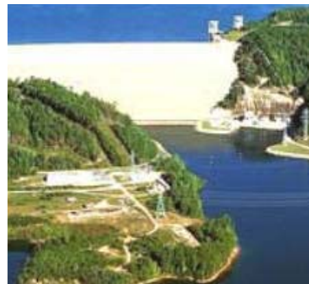
A pumped hydro facility
