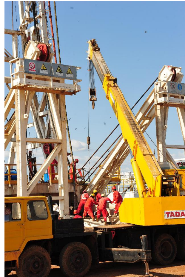
Project Site in Block 3/7, Sudan
