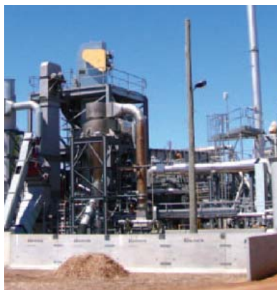
A biomass-fired power plant
