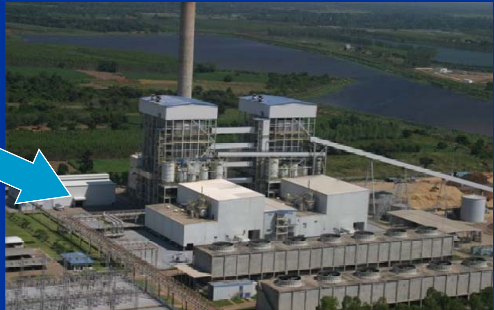
Biomass Power Generation
