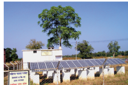
Stand-alone solar generation plant
